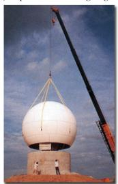
Strong, lightweight FRP/Composite domes use selfsupporting sandwich construction to protect sensitive electronic equipment from the Sahara to Antactica while remaining transparent to the electromagnetic signals.
